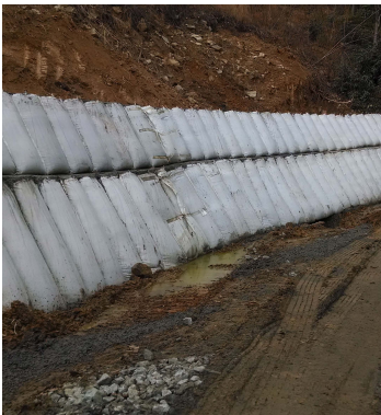
Roadside Levee Strengthening, KY
