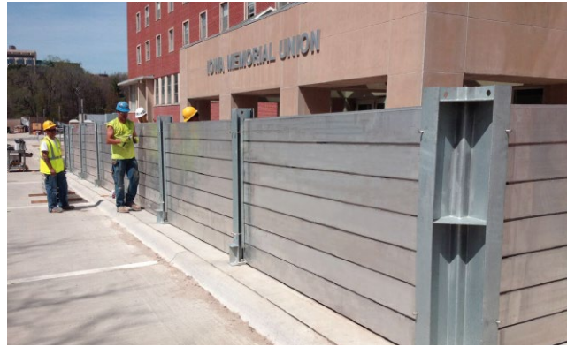
Corner Post Installation
