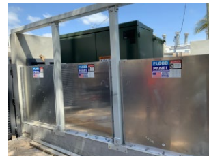
Custom support columns
