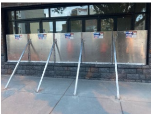
Vertical seam and support kickers
