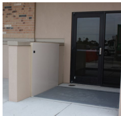
UTMB Primary Care Back Entrance, Galveston, TX
