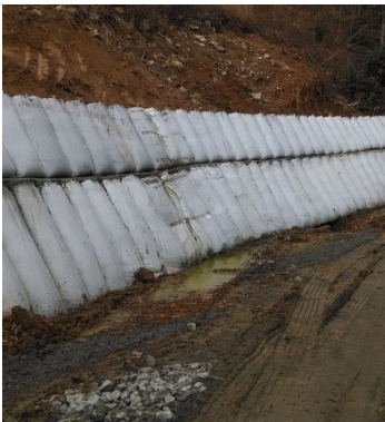
Roadside Levee Strengthening, KY
