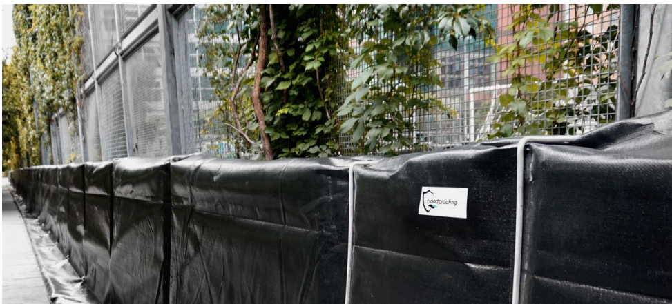
Muscle Wall Protecting Battery Park in New York City (Using Wrap Liner Option)
