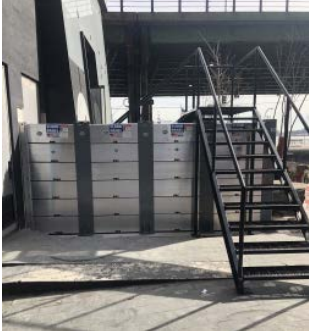
Emergency egress stairs
