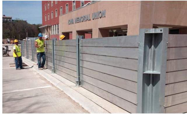
Corner Post Installation
