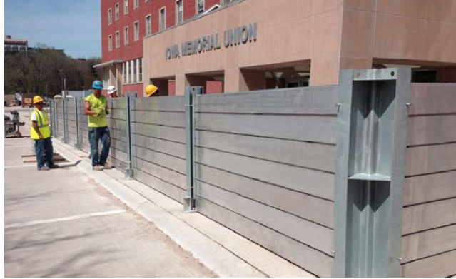
Corner Post Installation
