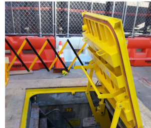
NYC Emergency Egress Hatch
