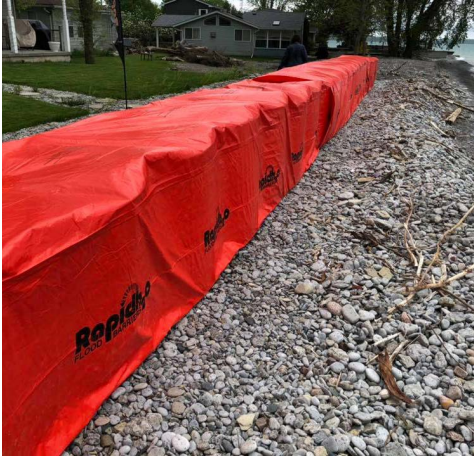
Protection From Shore Overflow
